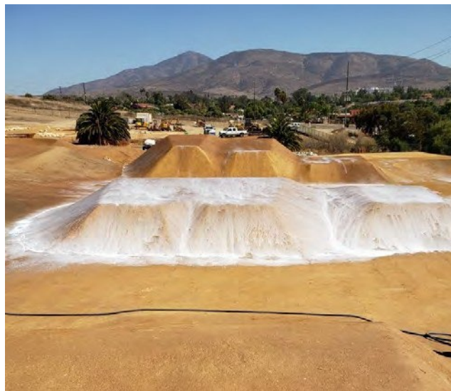
Soil Stabilizer Application - Sweetwater Bike Park
